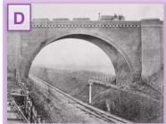
The lofty and well-built arches support the tracks of the Midland Railway. Originally a two-track railway, the join to the laterconstructed additional tracks can be clearly seen. Photo shows the earlier structure with branch line beneath. COURTESY ST ALBANS' MUSEUMS.
